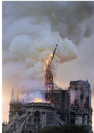
Flames and smoke rise as the spire on Notre Dame cathedral collapses in Paris, Monday, April 15, 2019. (AP Photo/Diana Ayanna)
